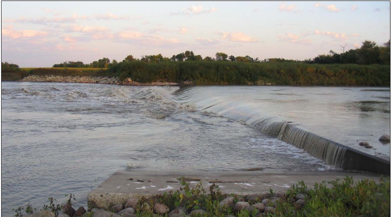
Figure 3. Drayton Dam on the Red River of the North, just north of Drayton, ND. Photo from September 18 th , 2008 at a river discharge of approximately 6,400 cfs.
