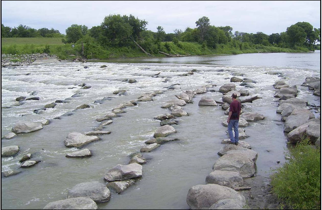
Figure 2. Example of a Red River fish passage project at Riverside Dam, Grand Forks, ND. Proposed project would generally look similar to this example.
