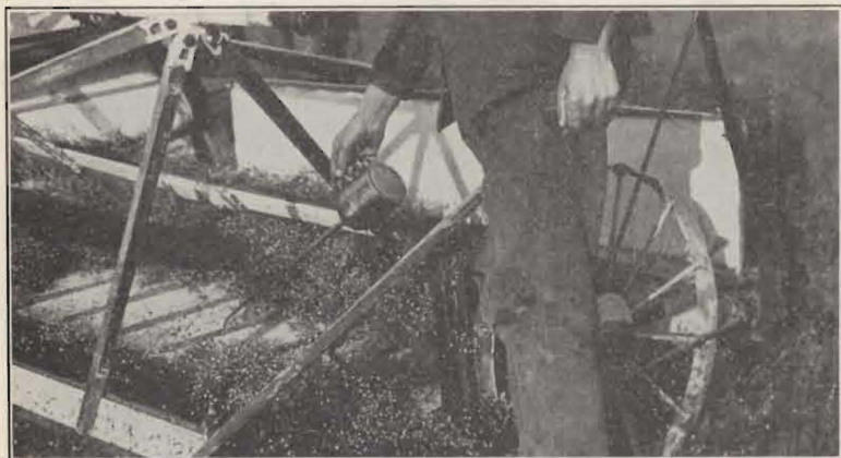
Fig. 21.—Green flax, or frosted flax, often tends to gum the sickle bars. This is easily remedied by applications of kerosene or gasoline.
