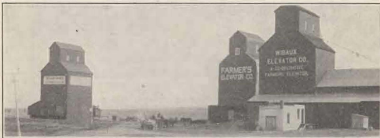
Fig. 33.—Rather typical western elevators into which the flax is dumped, showing farm teams, and cars being loaded for the Eastern market.
