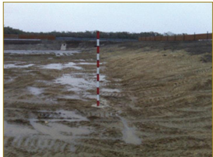
**Fig. 4. Installation of pond marker when the pond is empty or under construction**
