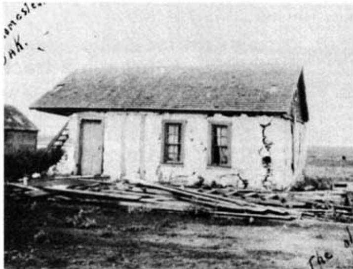
The first home of Adam Meidinger Jr. in Antelope Valley. It was constructed of stone and sod, measuring 12 ft. by 24 ft. The house was built in 1885. This picture was taken in 1946, at which time it was being torn down.
