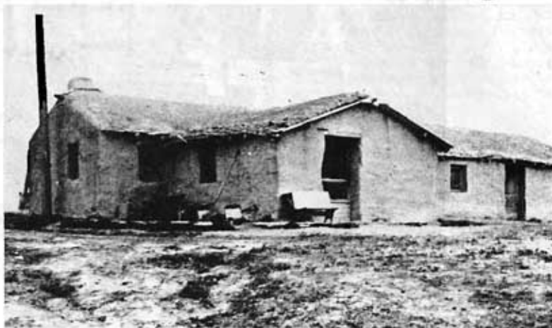
A stone and clay structure with clay roof and "bee hive" type of chimney. The picture appeared in "Russian-German Settlements in the United States."
