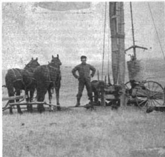
Horse-powered well-drilling scene in early 1900s in North Dakota's McIntosh County. The mud cart which one of the men has in his hand is made with buggy wheels.
