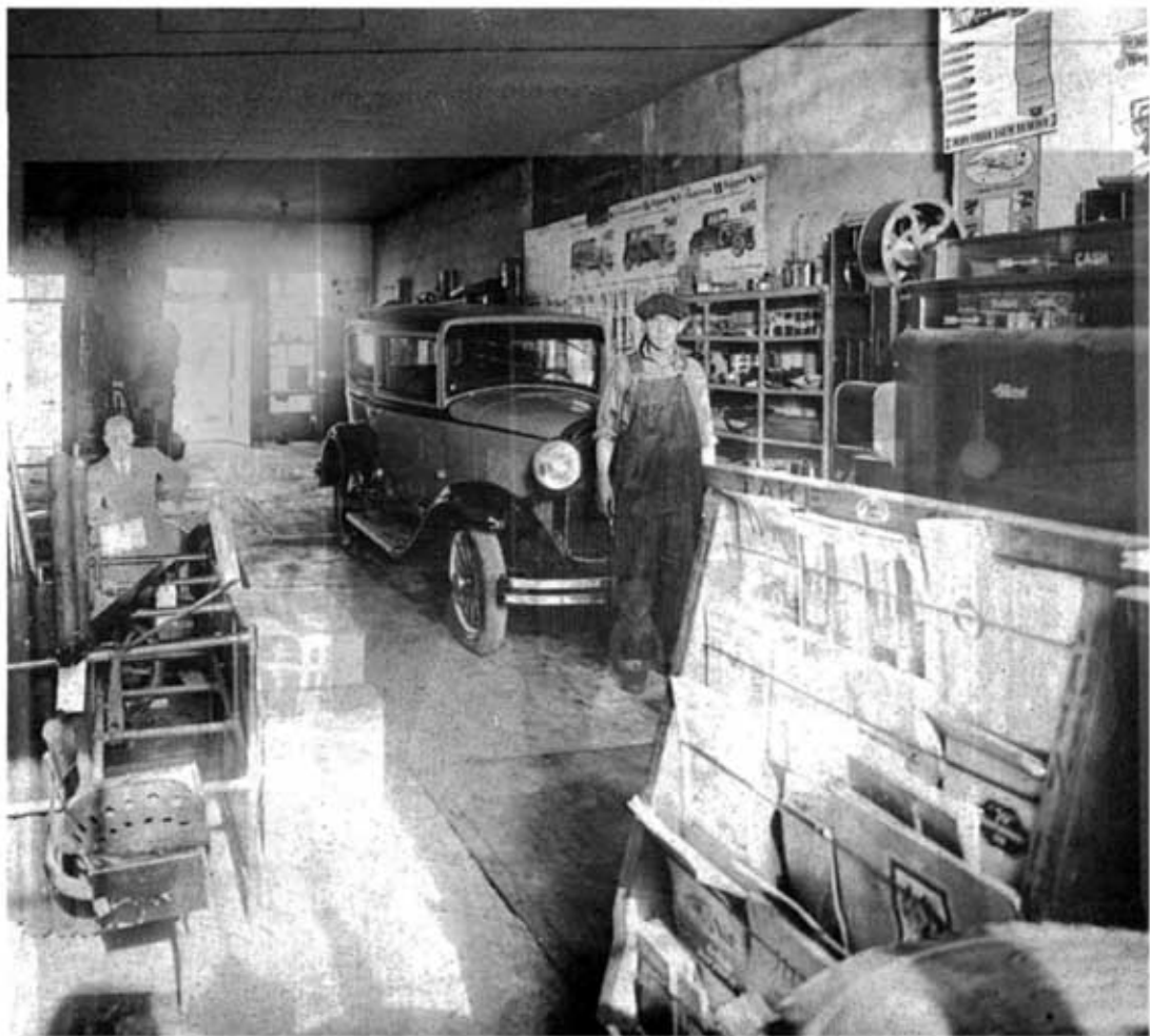
Gerald Bailey is standing by a new car in the John Pudwill Garage in Wishek. Pudwill sold Overland and Whippet cars. The building was located where the Wishek senior citizen building now stands.
