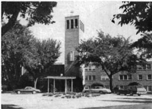
F rom humble beginnings to a modern complex built in red brick: Presentation Heights in 1985.
