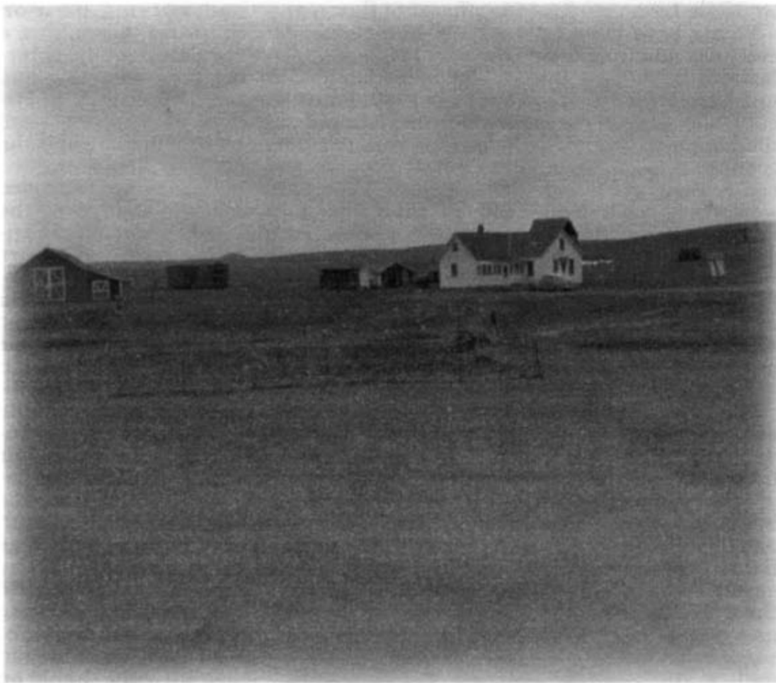
The farm, which is easily seen from the highway near the Morton/Mercer County line, is shown in the latter days of the farm after the framed house was built in 1908.
