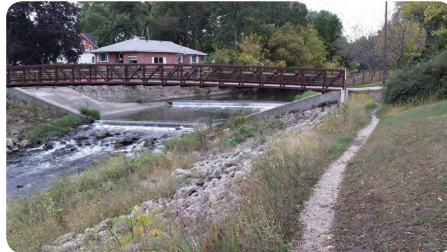
Above: Manmade weirs used as flooding control.
