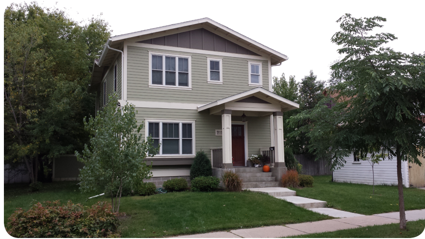
Figure 2.2: The first house to be built in Kutzky Neighborhood in over forty years. (Photo Credit: Josh Wildt, October 2013)
