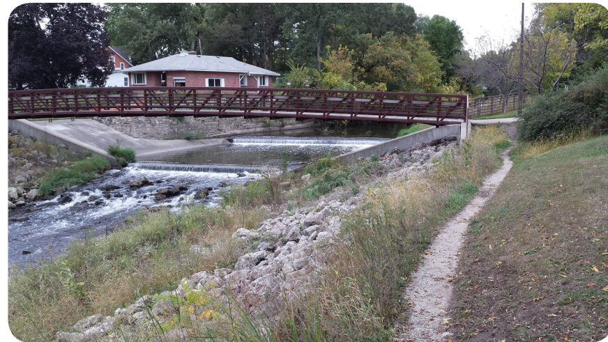
Figure 3.11: Existing flood prevention along Cascade Creek right before entering the Zumbro River (Photo Credit: Josh Wildt, October 2013)
