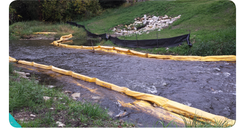
Figure 1.1: Example of existing conditions at Cascade Creek. (Photo Credit Josh Wildt, October 2013)
