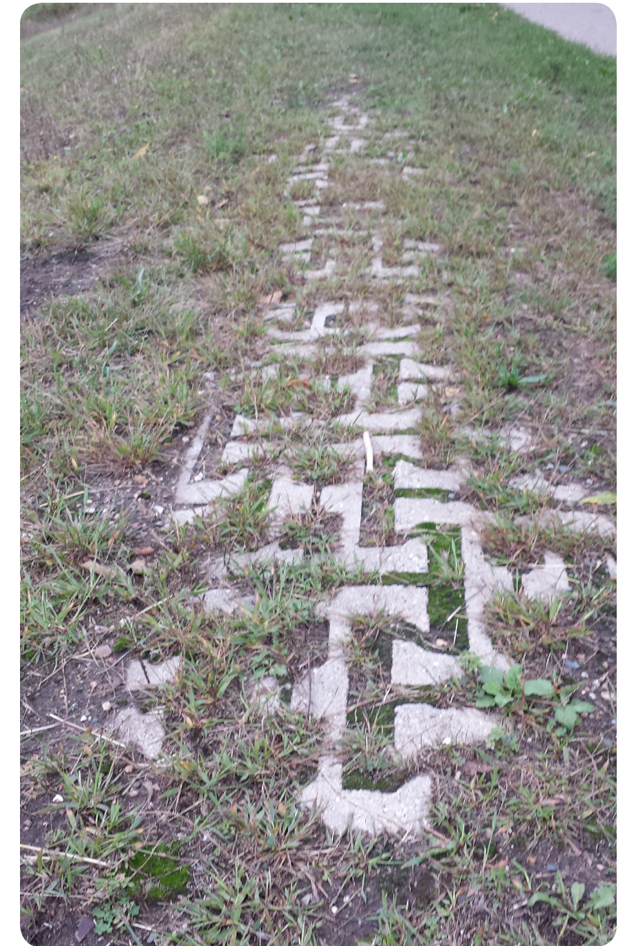
Figure 3.9: Another example of a riprap bank. (Photo Credit: Josh Wildt)
