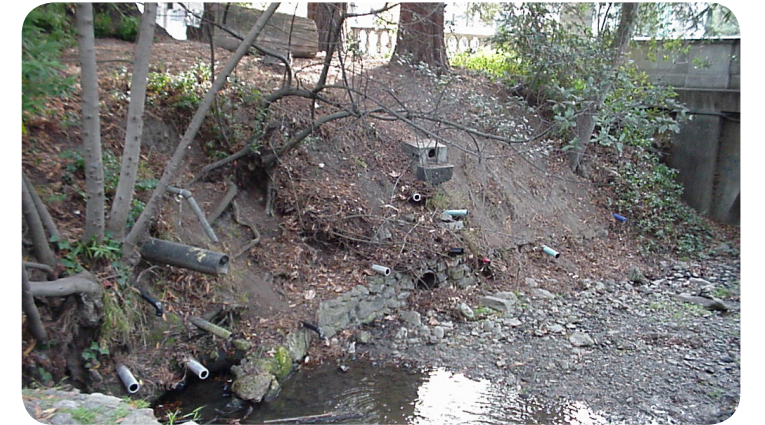
Figure 1.6: Existing conditions along the creek (Photo Credit: UC Berkeley)
