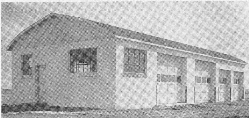
FIGURE 7.—This shop building, with vehicle storing space, can house three vehicles, additional equipment, plus its well-equipped workshop area.
