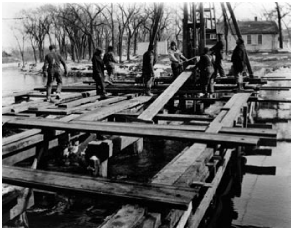
Constructing 4th Street dam, Fargo, 1930. (IRS, NDSU, Fargo, 2022.4.1.
