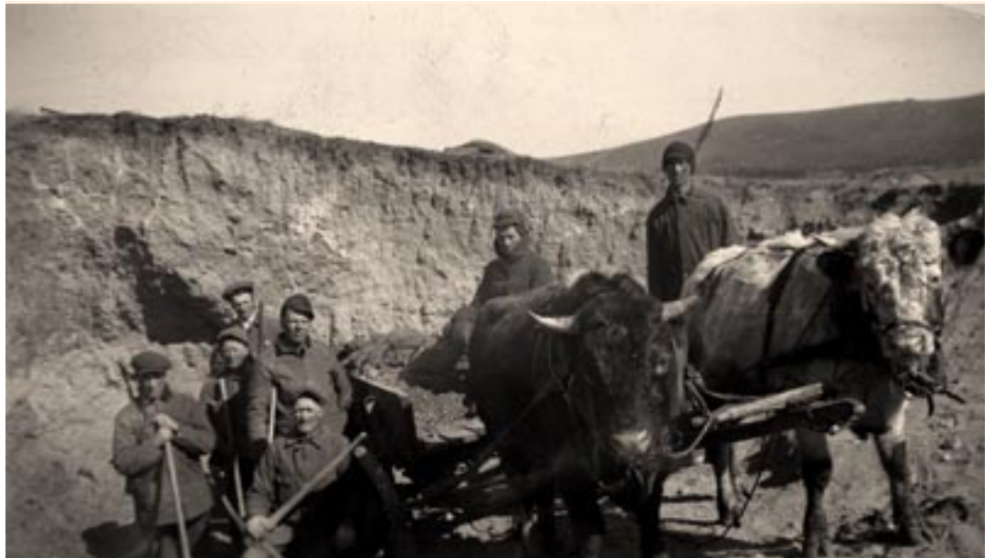
Works Progress Administration (WPA) project in the 1930s. (IRS, NDSU, Fargo, Mss 296.205.1)
