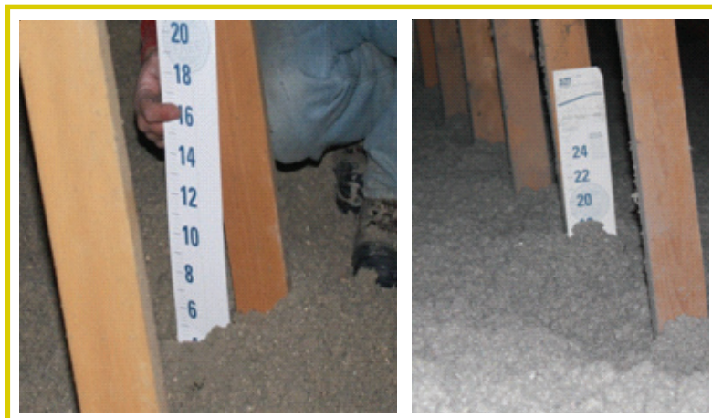
Attic insulation, before and after.
