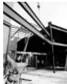
Workers place last beam on Minard addition
