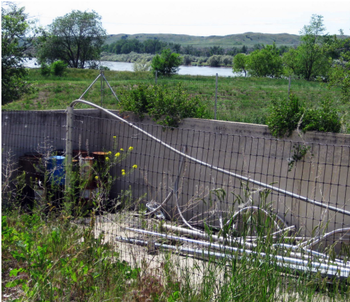
Empty Water Tank
