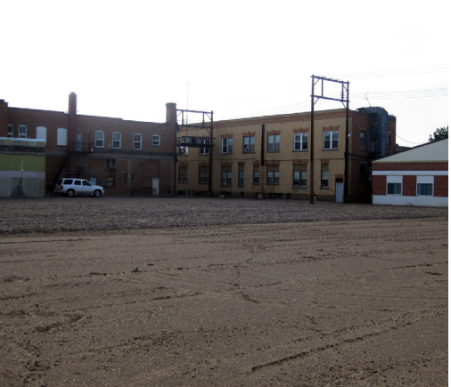
View from SE corner
