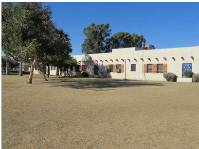
A SMALL PRIVATE SCHOOL NEIGHBORING THE OFFICE BUILDINGS TO THE WEST.
