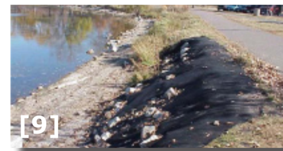
Phase 2 - Shoreline Stabilization
