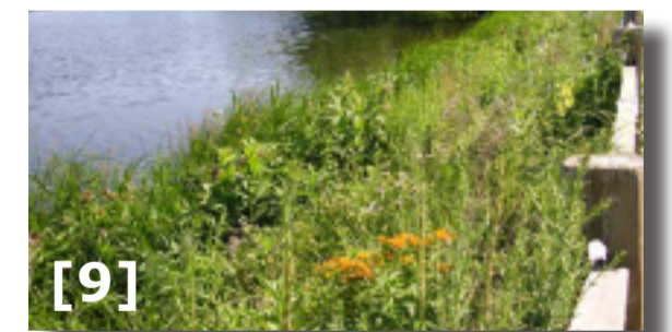
Phase 3 - Shoreline Restoration
