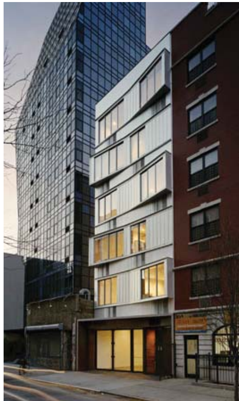
All Switch Building images from: Architectural Record; June, 2008
