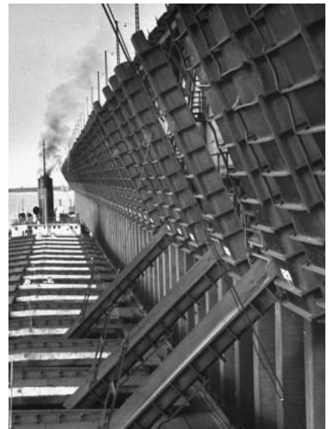
taconite being loaded
