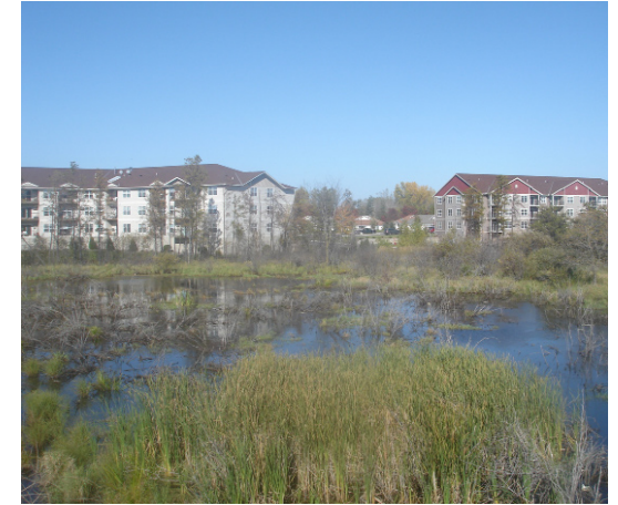
Picture owned by Erik Twistol Apartment building to the East of the trail.
