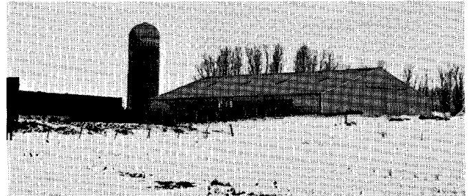
SILo location near the feeding area minimizes hauling and conveying time. Provide for filling access from the service yard.
