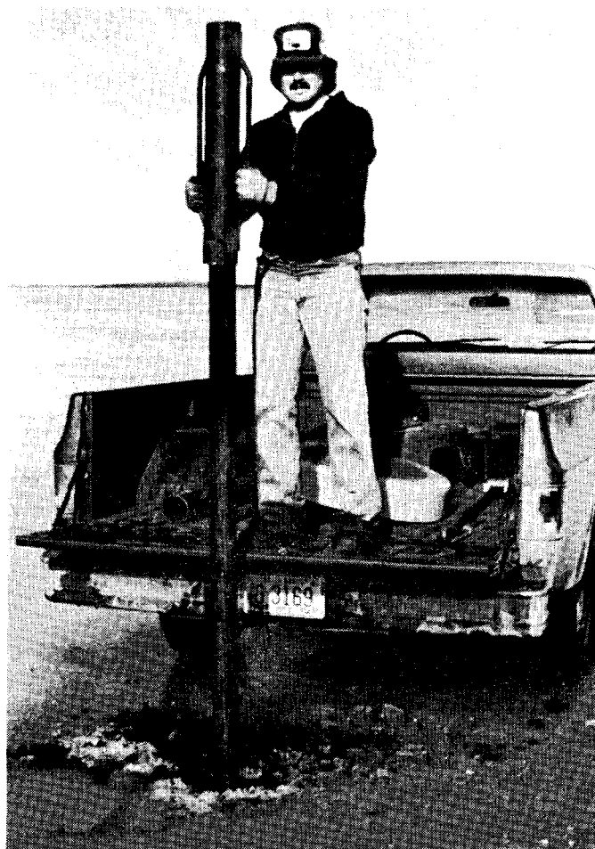
Figure 11. The best time to begin installing nesting structures is in December once the ice is thick enough to support people and equipment. (G. Enyeart)
