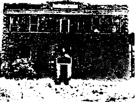
4. Abandoned brick school presents danger.
