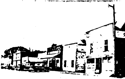
1. One dilapidated building can spoil your downtown.
