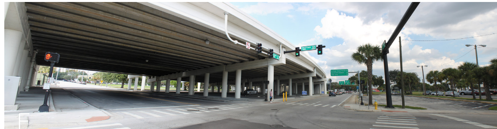
(Figure 45, Site View F)
