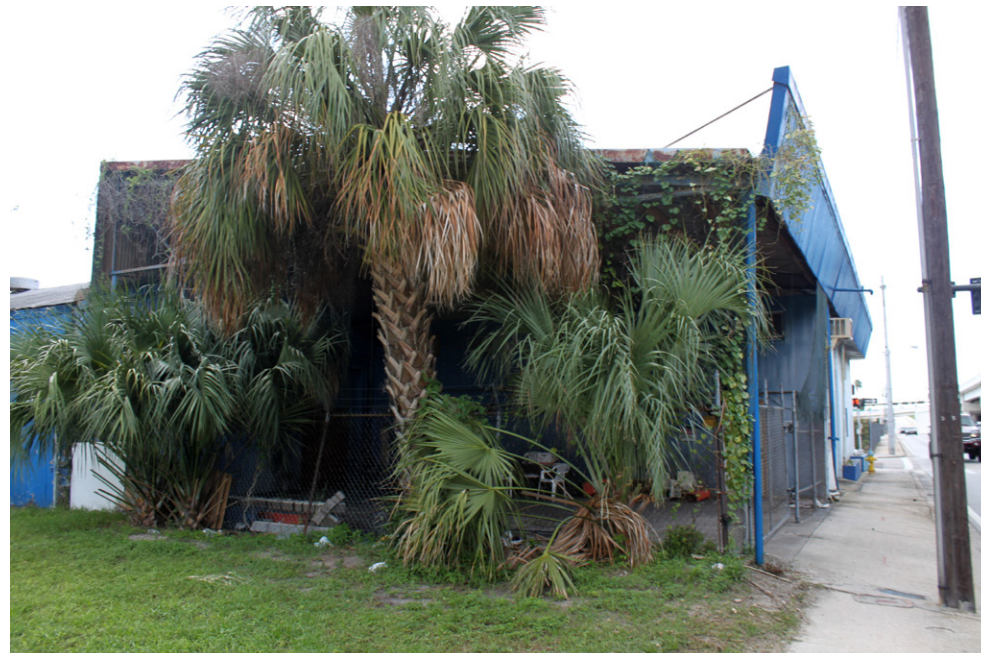
(Figure 22, Abandoned Building)
