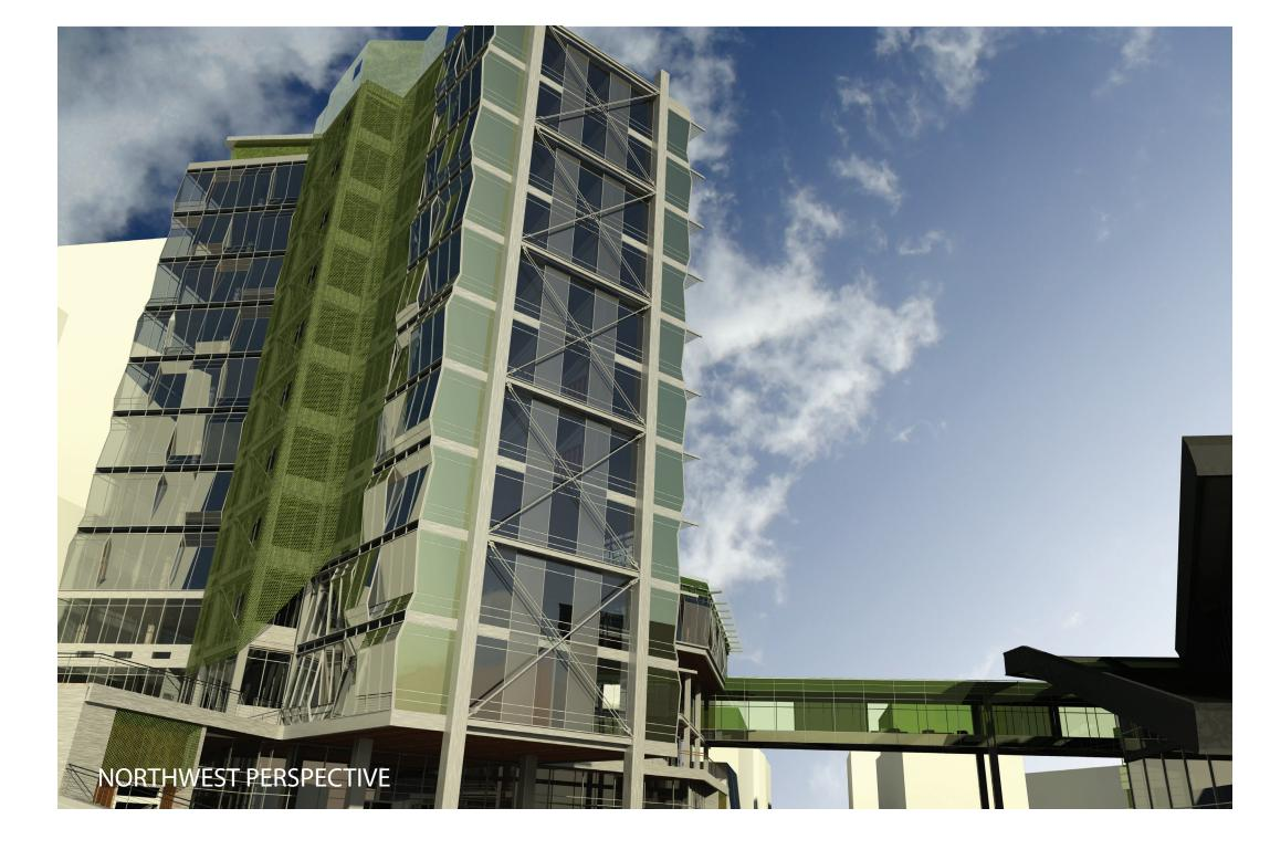
Glazing details that promote autonomy: the undulation of the glass within the units allow for a greater field of view than typical perpendicular glazing. Not only are views increased up and down, but also side to side.
