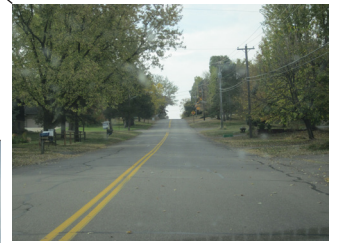
Well-traveled road that has no place for pedestrian travel.
