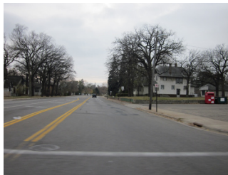
Wide residential road with a sidewalk right next to the street.
