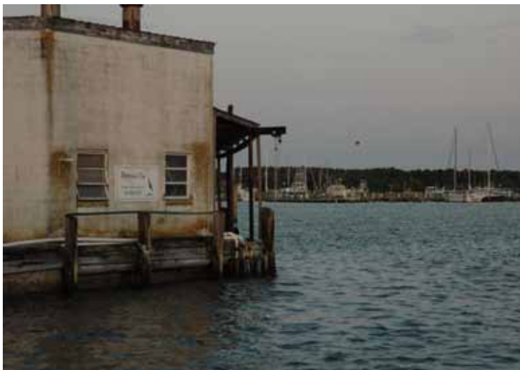
Photo courtesy of: Travis Steffen
