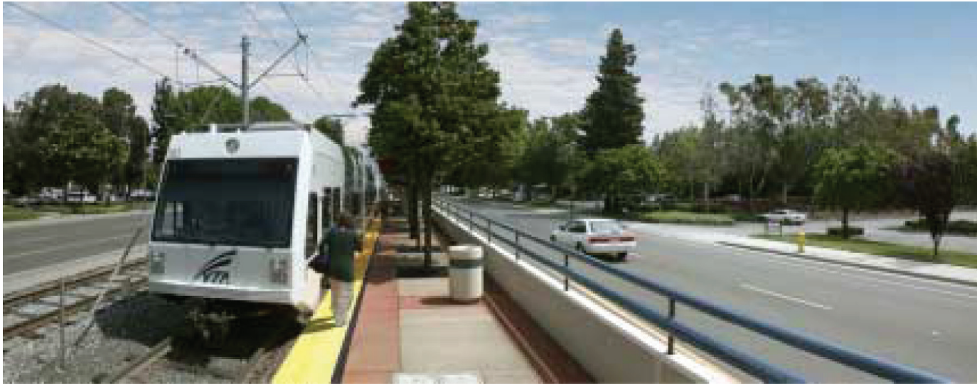
North First Street: Before and After
