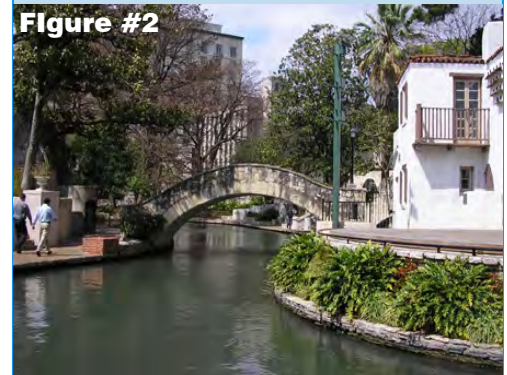
Figure #2 A series of bridges along the paths allows for easy access to the other side of the river.
