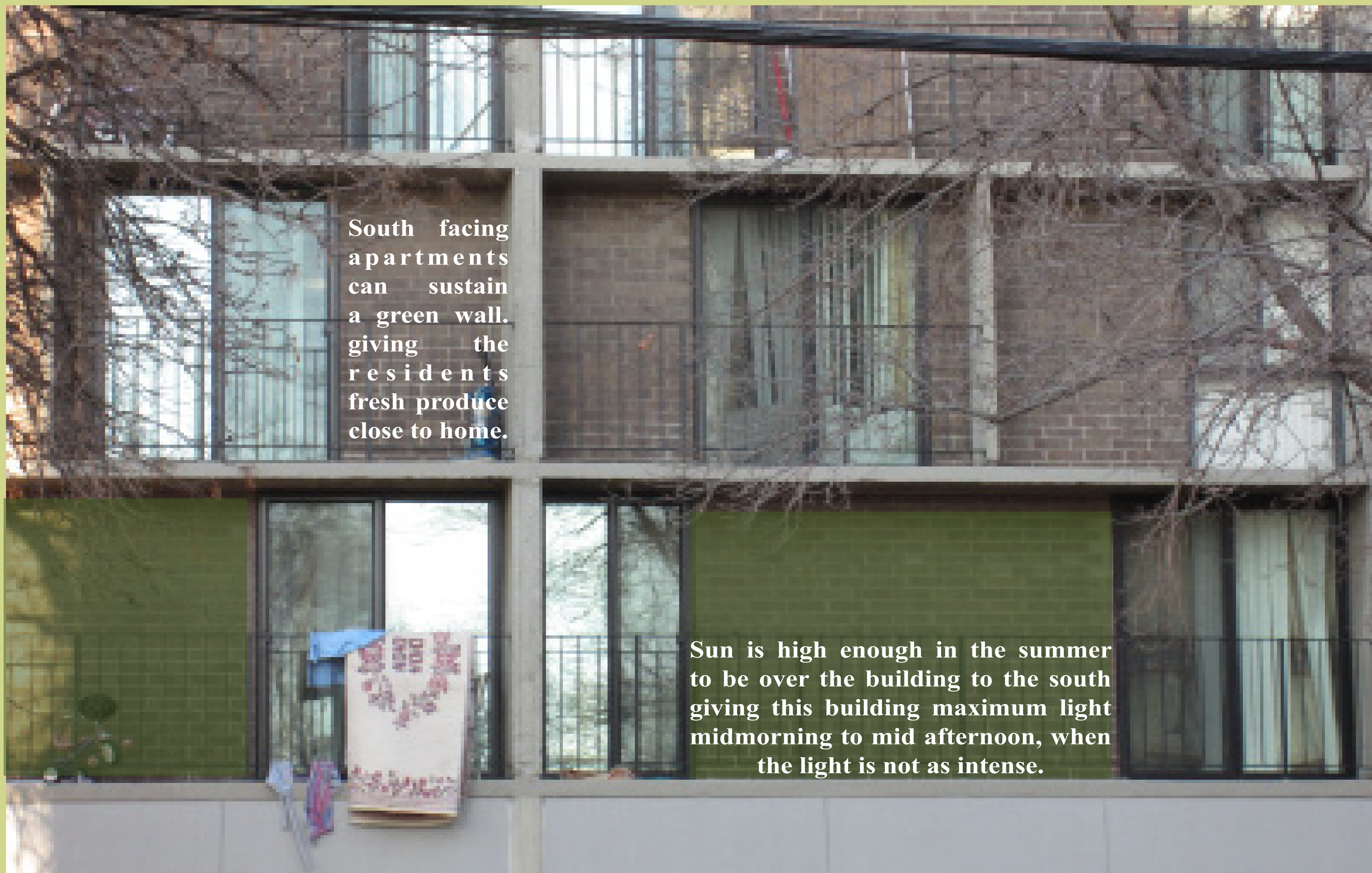
Above is an analysis of the sun in relation to the building orientation. The buildings are oriented with the apartment windows facing south or southwest, which will give them optimum sunlight for growing.
