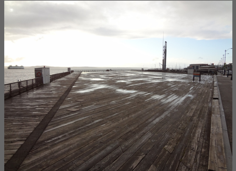
facing northwest on pier 62/63
