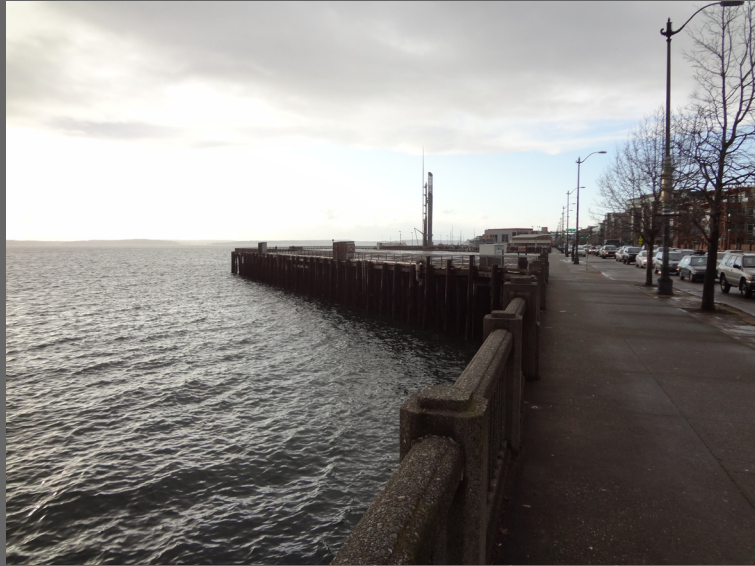
facing north toward pier 62/63
