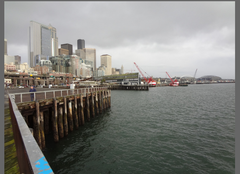
facing south east toward pier 62/63
