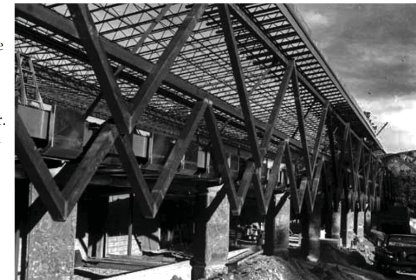
FIGURE 12 Beaver Meadows Visitor Center Under Construction in 1966 (Lockwood)
