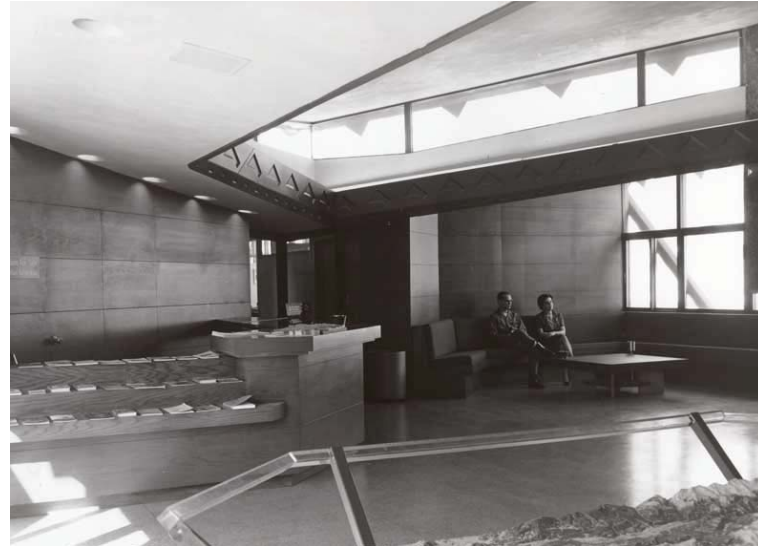
FIGURE 17 BMVC Lobby 1967 (National Park Service)
