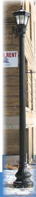
Lighting Poles in the neighborhood
