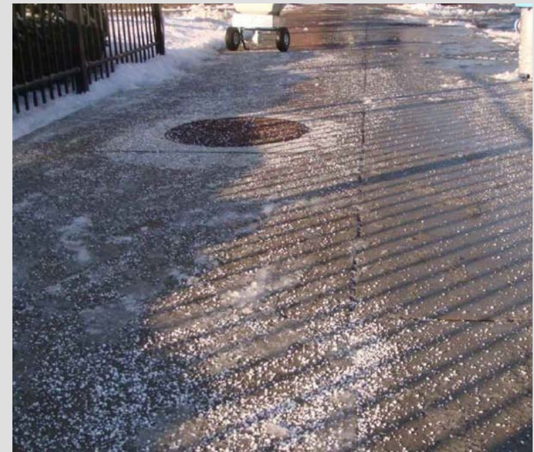
Figure 11. Salts poured on roads and sidewalks to melt ice and snow during the winter. (Source: http://www.alibaba.com/product-gs/439884022/Ice_Melting_Salt_for_Road_96.html )
