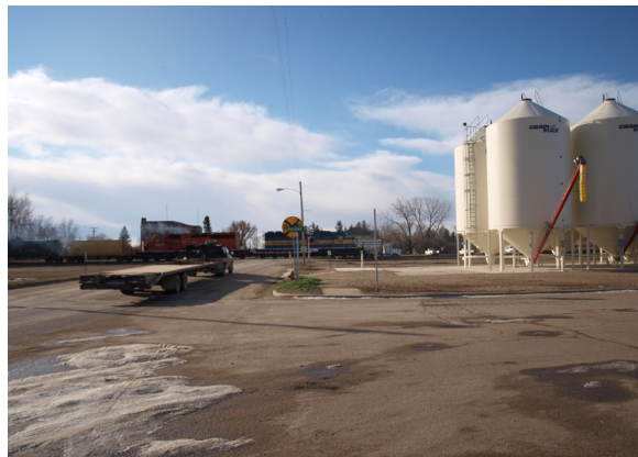
Top Left: The top of the SunPrairie Grain elevator which stands 128 feet high. Left: Train engines from the Canadian Pacific Railway pass by the railroad crossing next to the project site.
