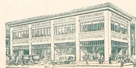
STONE BUILDING 826-828 Nicolet Ave., Minneapolis, Minn.
