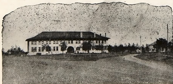
Francis Hall, When It Was the Old Dormitory.
