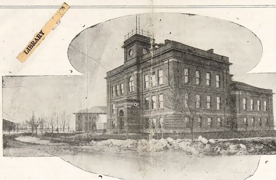
Chemical Building which was entirely destroyed by fire on the night of December 24th.
