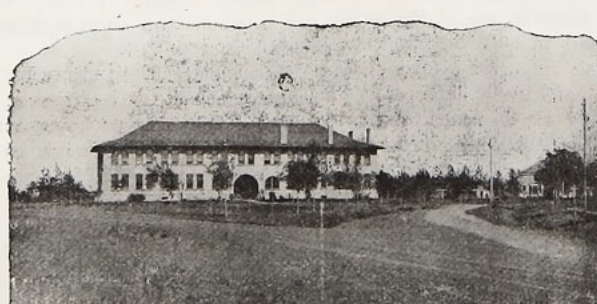
Francis Hall as the "Dormitory".
