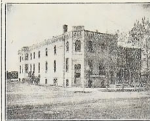
The largest and most modern Creamery Building in North Dakota.
