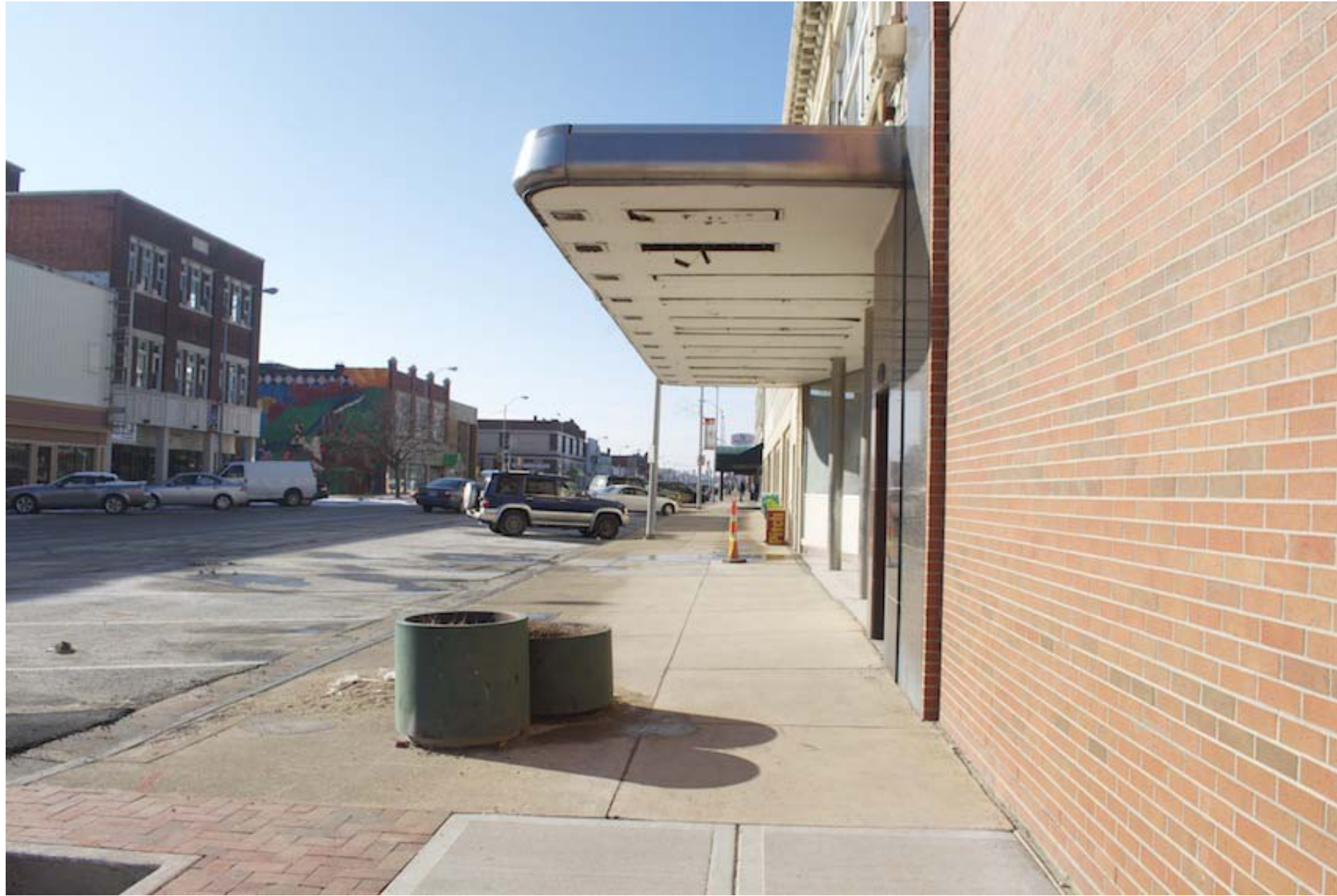
Lack of uniformity in the sidewalks on Minnesota Avenue
