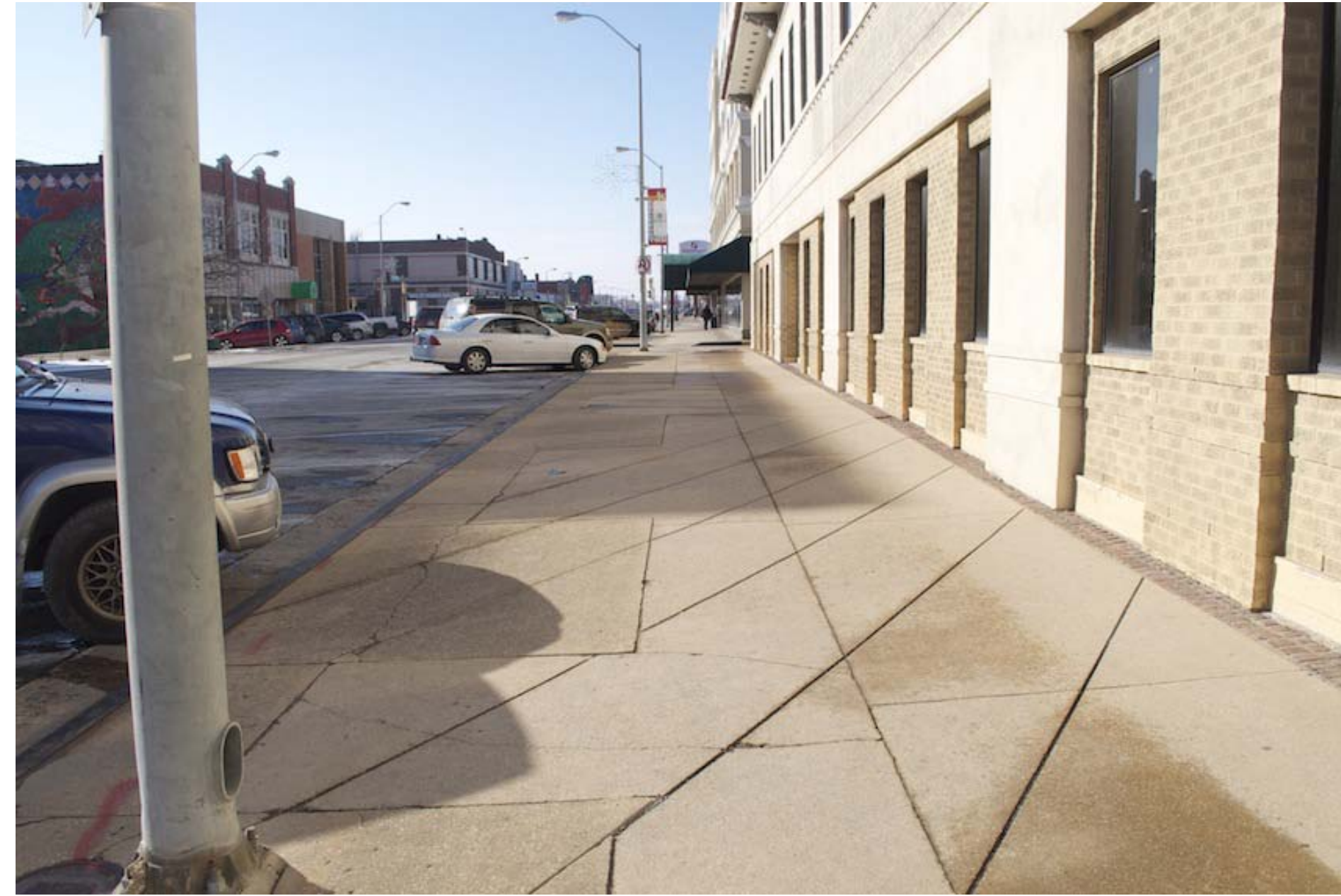
Large sidewalks with no purpose
