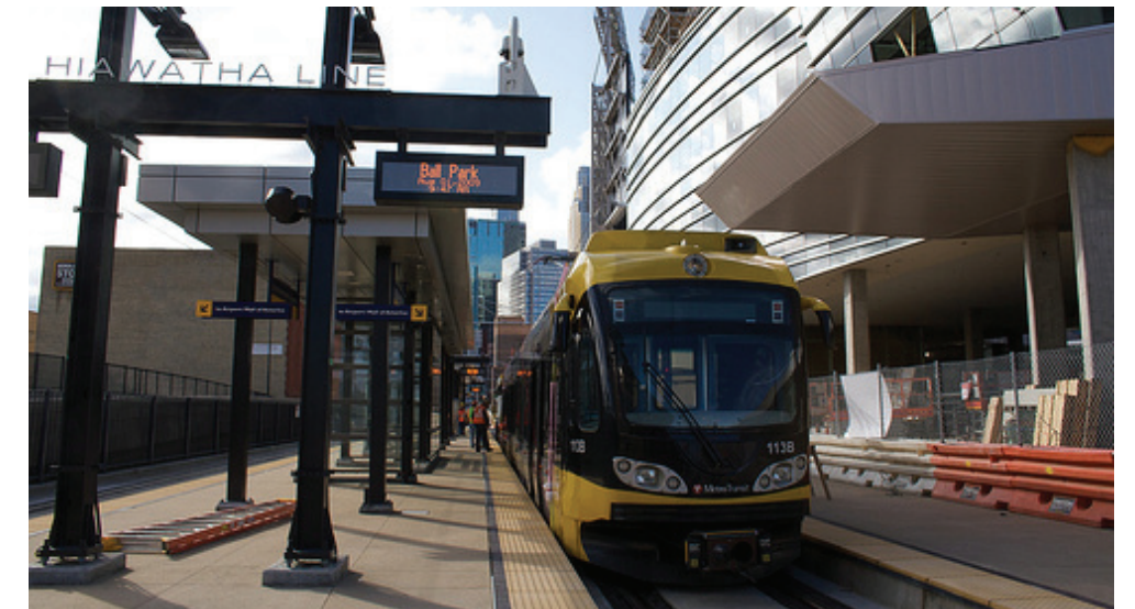
Figure 3.2. Transit station on the Hiawatha Lane. Retrieved from http://northstar.typepad.com/northstar_commuter_rail/2009/08/august-8th.html
