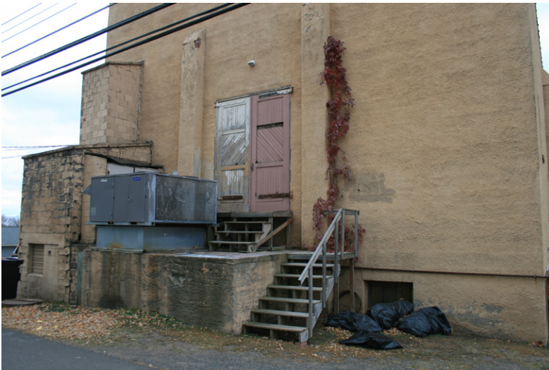
textures on back of existing theatre
