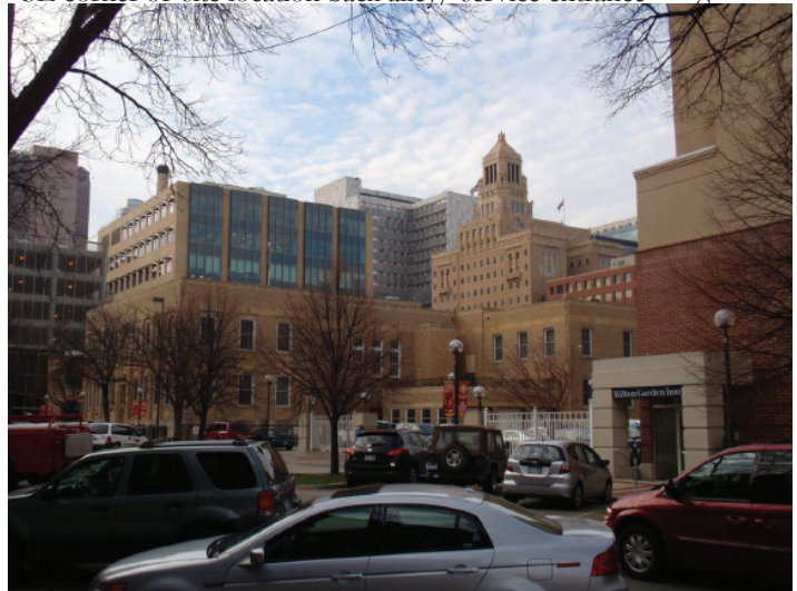
SE corner of site location back alley/ service entrance Figure 42
