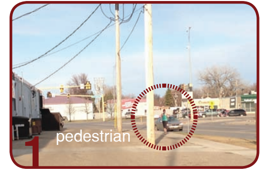
Existing sidewalk condition
