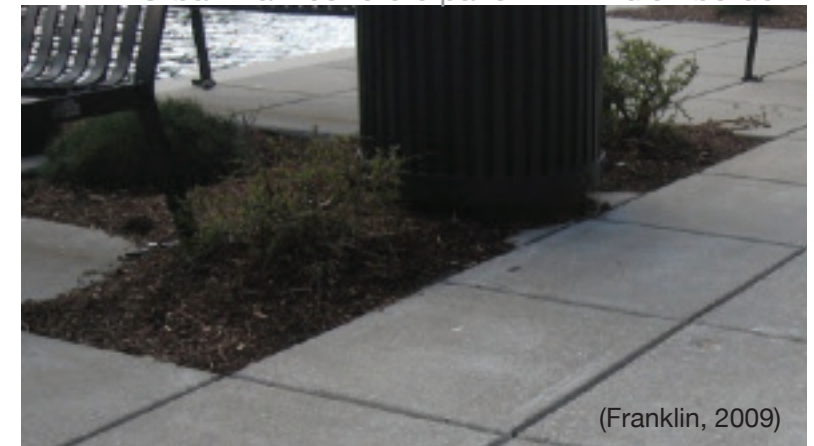
Urban trail: cast scored concrete with plantings
