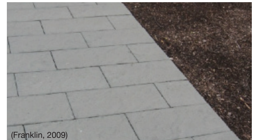
Urban trail: concrete paver with mulch border
