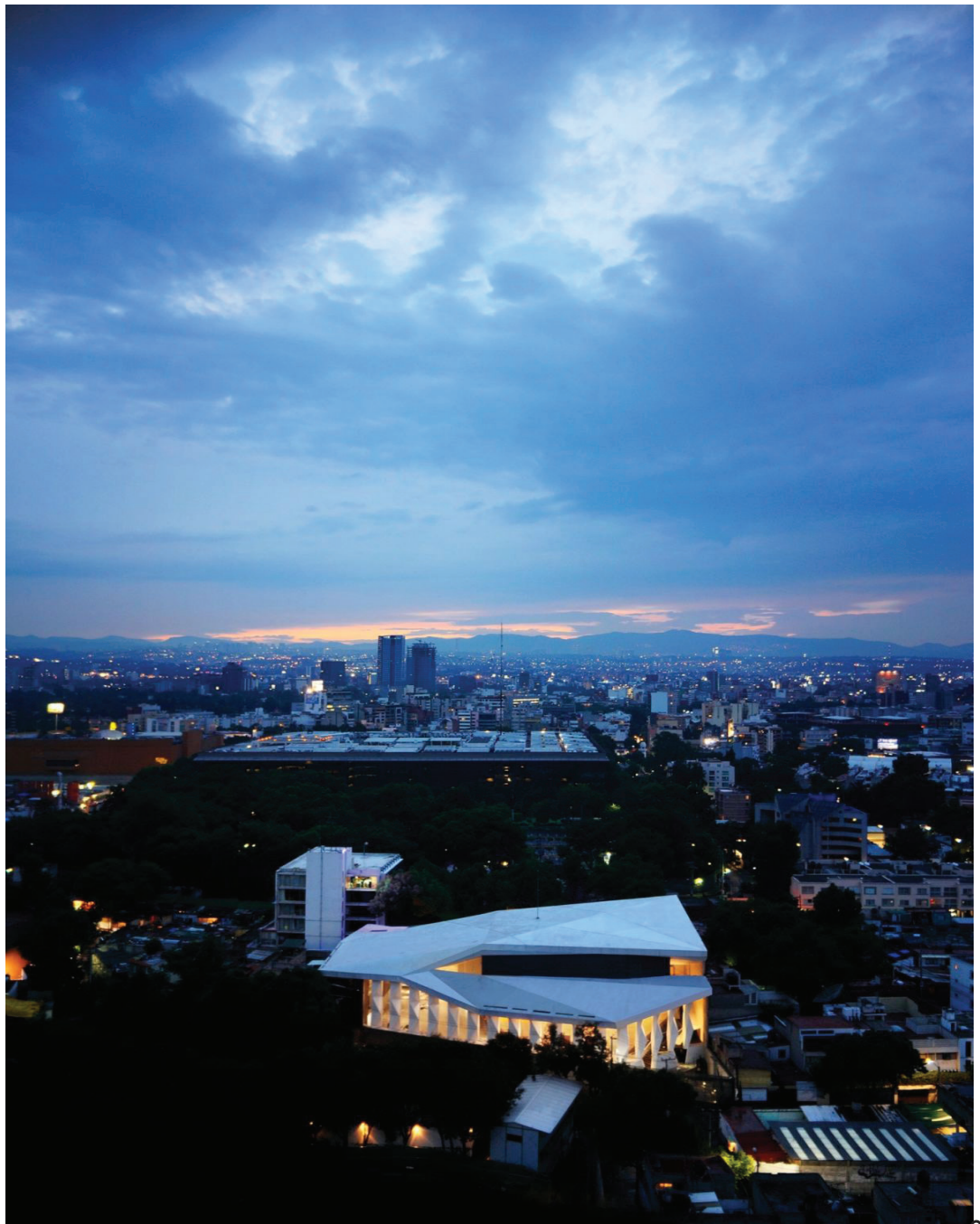
EXTERIOR VIEW FIGURE 27
