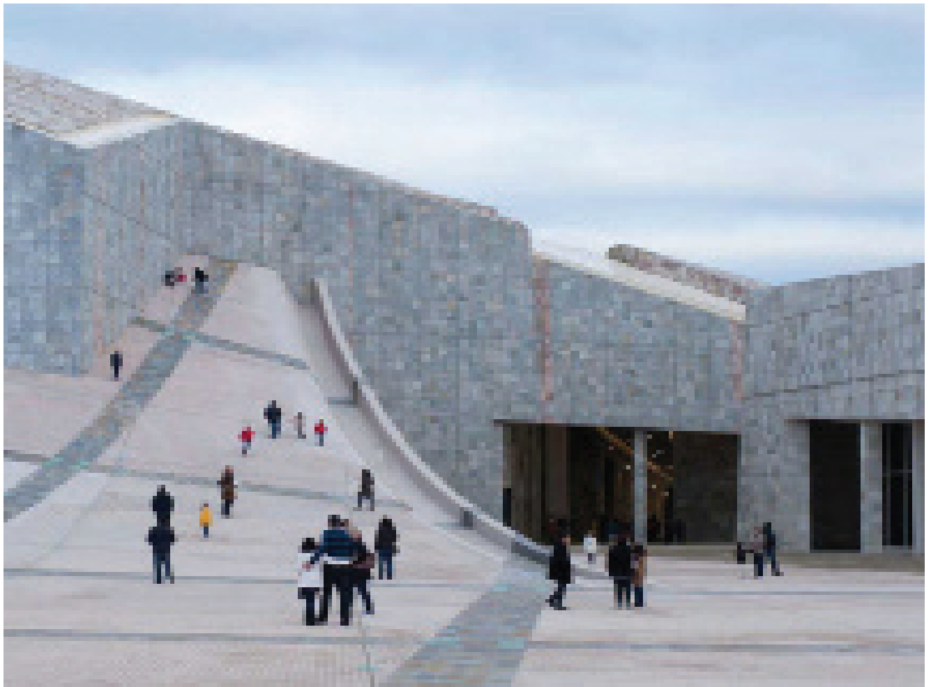
EXTERIOR VIEW FIGURE 13
