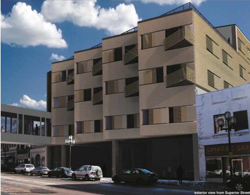
exterior view from Superior Street
