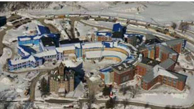
Worcester Recovery Center and Hospital | Aerial photograph of construction | (Mass.gov 2012)
