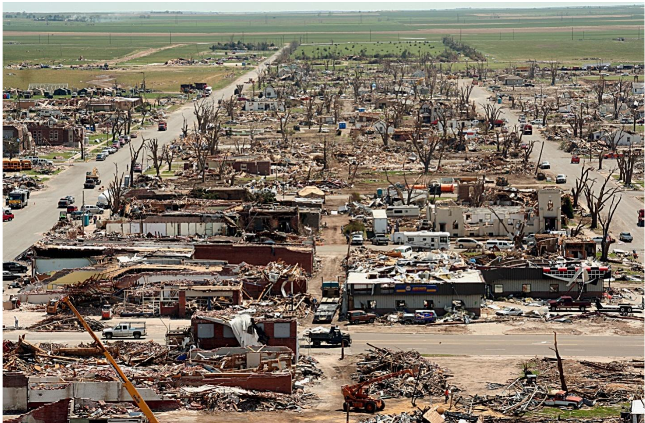
Figure 7. Greensburg Kansas damaged (Source FEMA, 2012 http://www.photolibrary.fema.gov/photodata/original/30066.jpg ).
