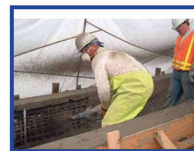
Figure 82 -“Fig 7: Formwork and finishing screeds (plastic pipes) installed” (American Shotcrete Association, 2008, p.39)
